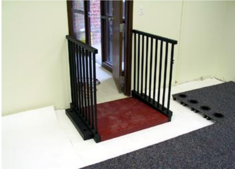
Rails located both sides of ramp
