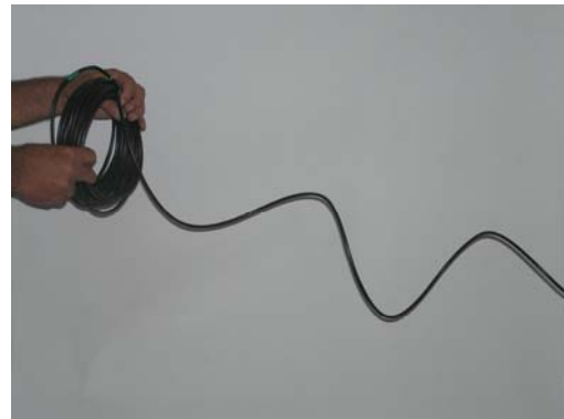
Wrong !!! Pulled off the coil and pulled straight, will result in damage to the cable.
