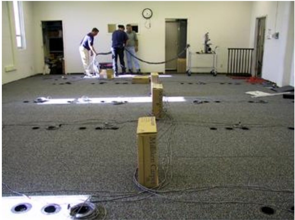
Rolling Out & Sorting Cabling on Top of Floor
