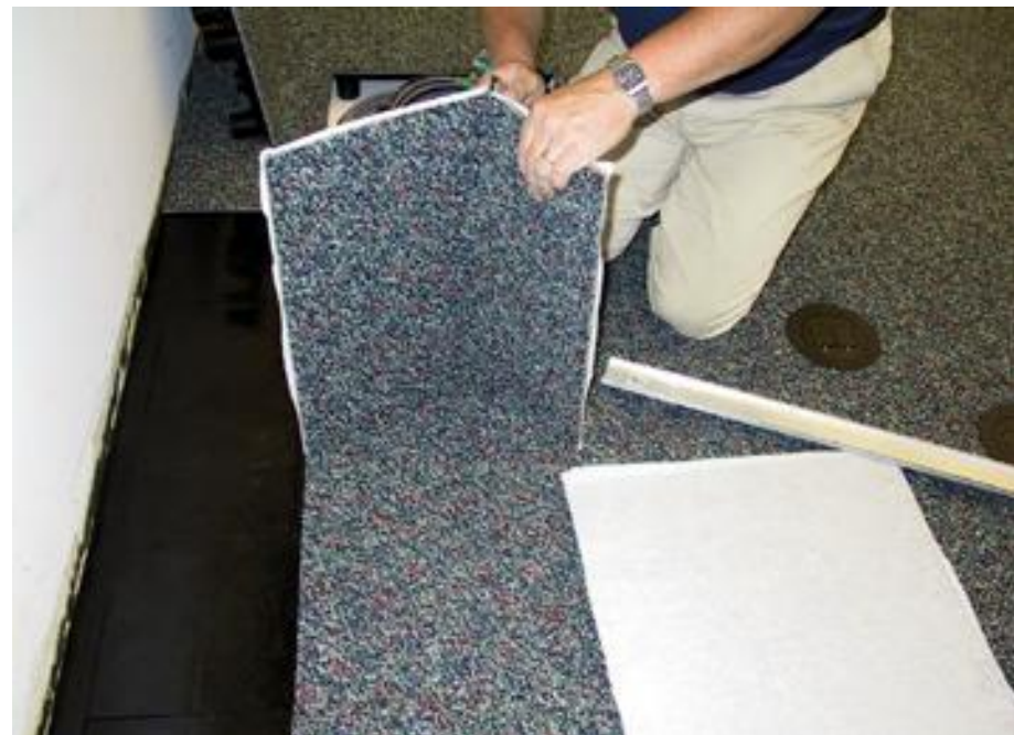
Cutting carpet tile for perimeter
