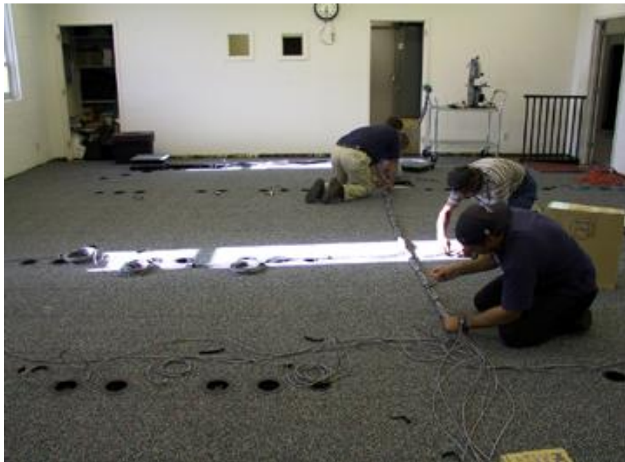
Tie Wrapping as Required
