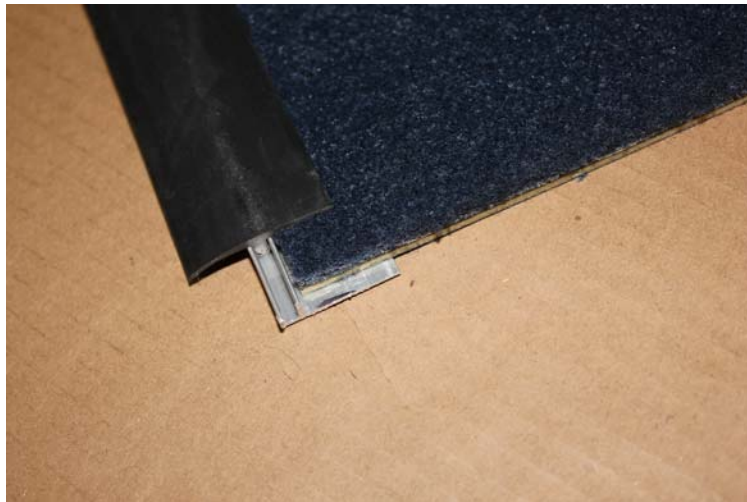
Transition Molding completed
