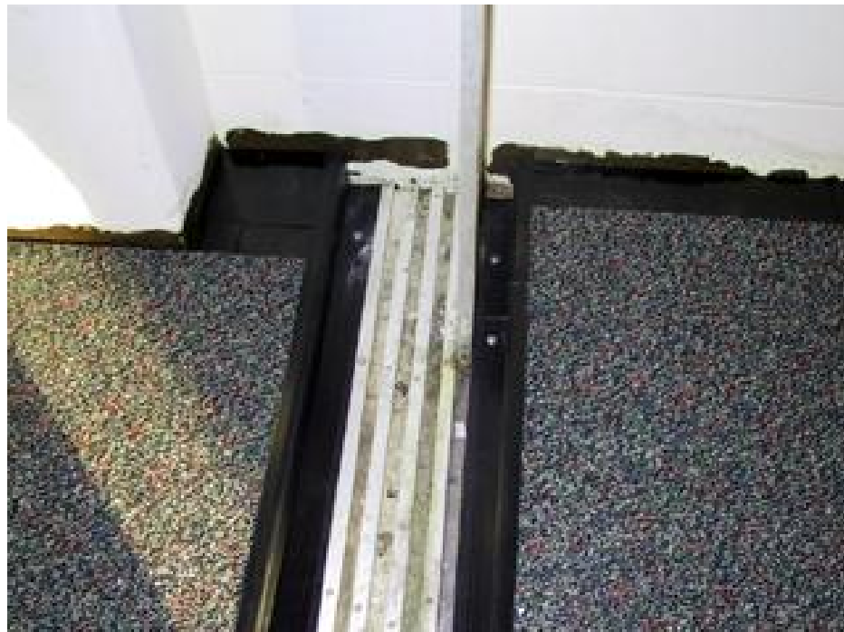
Picture 7-15 Z Trim Installed
