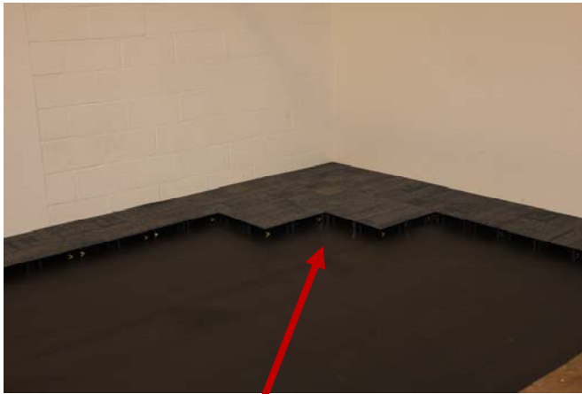
Picture 5-2 Installing Foam Underlay
