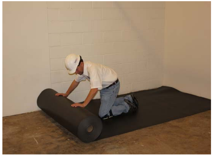
Picture 5-1 Foam Rolls / Installing Foam Underlay
