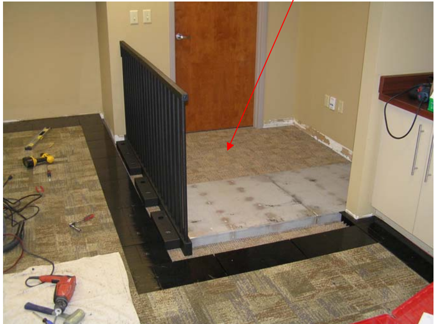
Drilling Ramp for countersunk anchors
