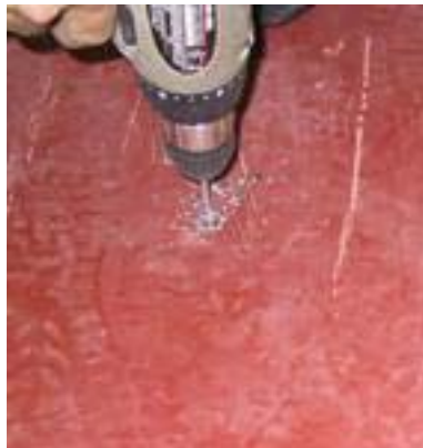
Drilling Ramp for countersunk anchors
