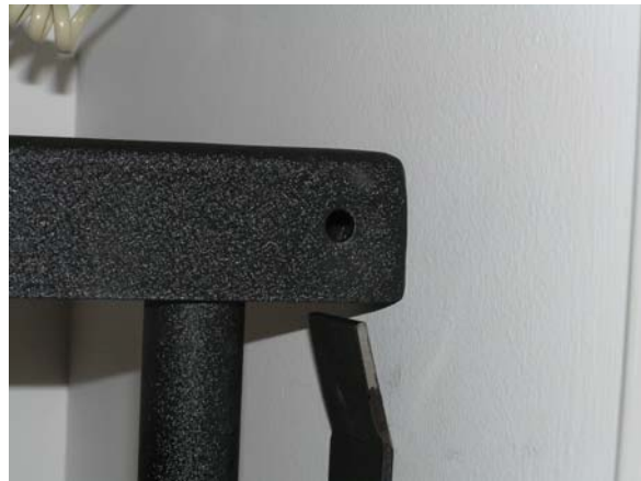
Rail Top Cap Hooks on Wall Bracket
