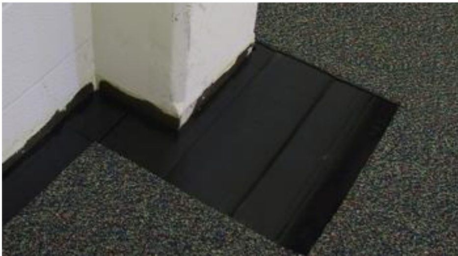
Filling in Perimeter around obstacles
