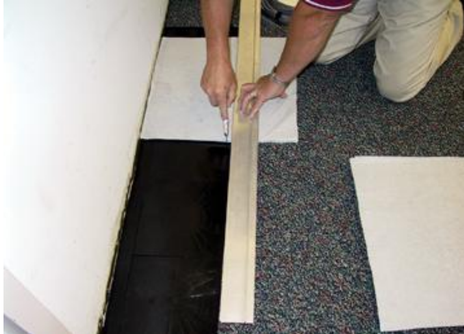
Cutting carpet tile for perimeter
